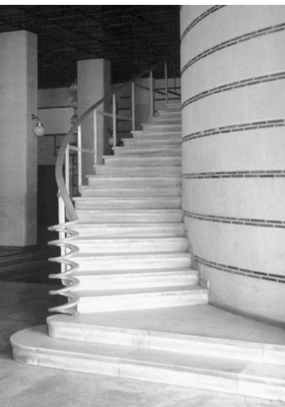
Figure 6 Stair detail, Faculty of Languages building.
